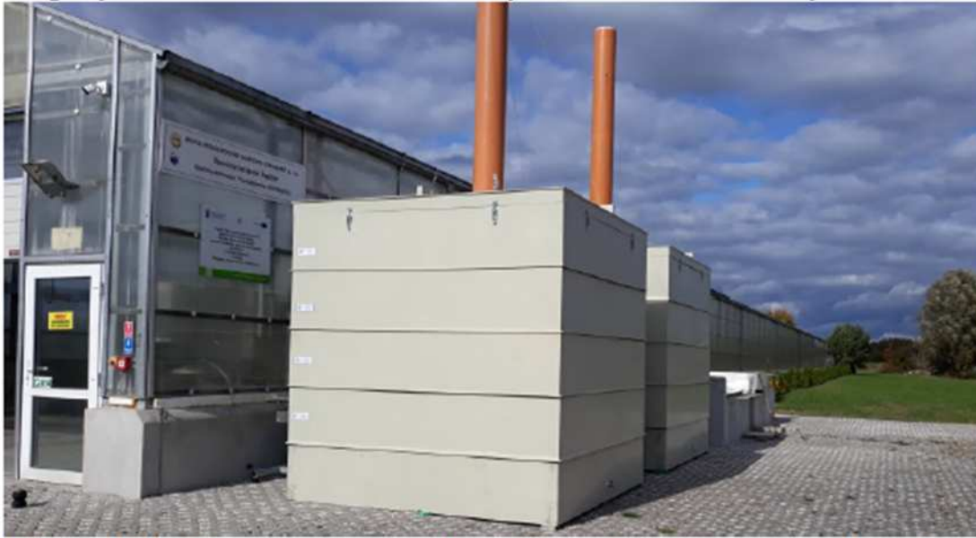
Fig. 3 Biofilters with Halosorb bed operated in a WWTP
